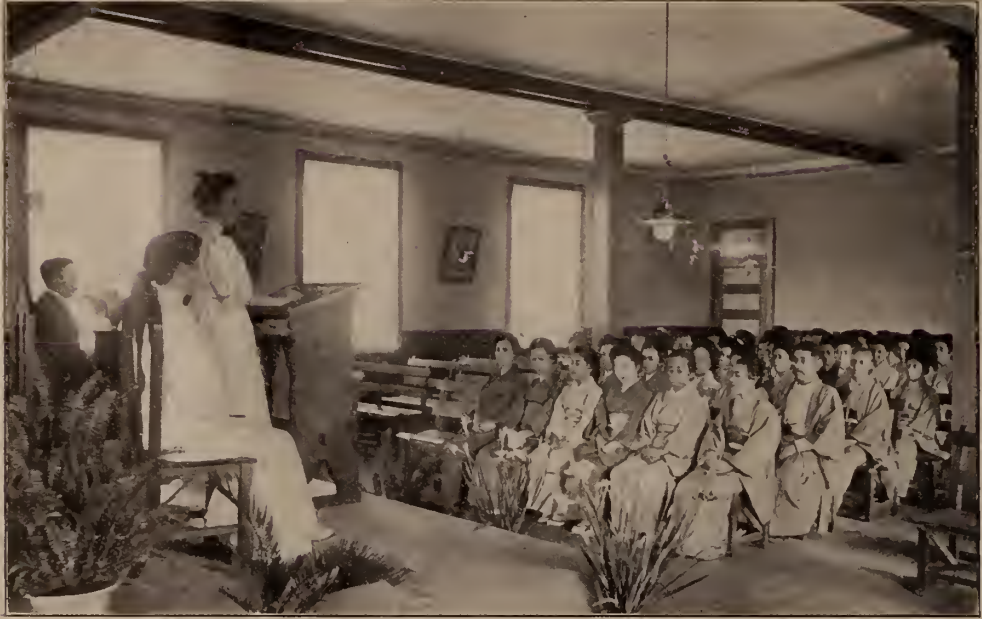
INTERIOR OF PIERSON CHAPEL.
